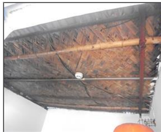
Photo of non-conformity Flammable Ceiling.JPG
