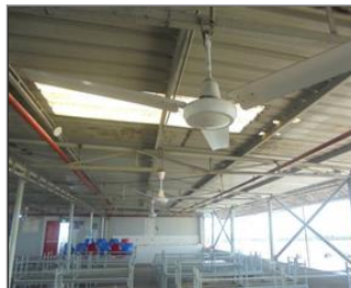
Photo of non-conformity Low height overhead fan.JPG
