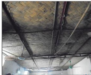
Photo of non-conformity Overhead flammable ceiling.JPG
